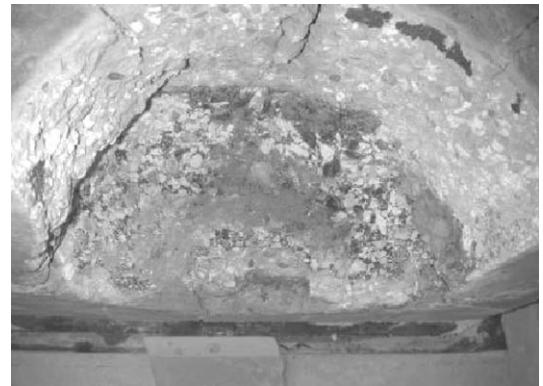
Fig. 12. Post-test view of the concrete cavities for VB-U6 (limestone-rich concrete G).
